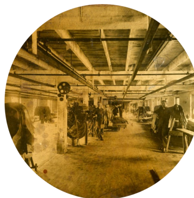
A023.14.224—split finishing inside Robson Tannery.
